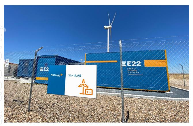
Figure 1 E22 250kW/675kWh VRFB installed in Zamora, Spain
